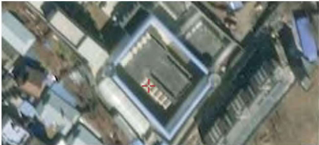
Figure 93 - Dazi County Detention Center
