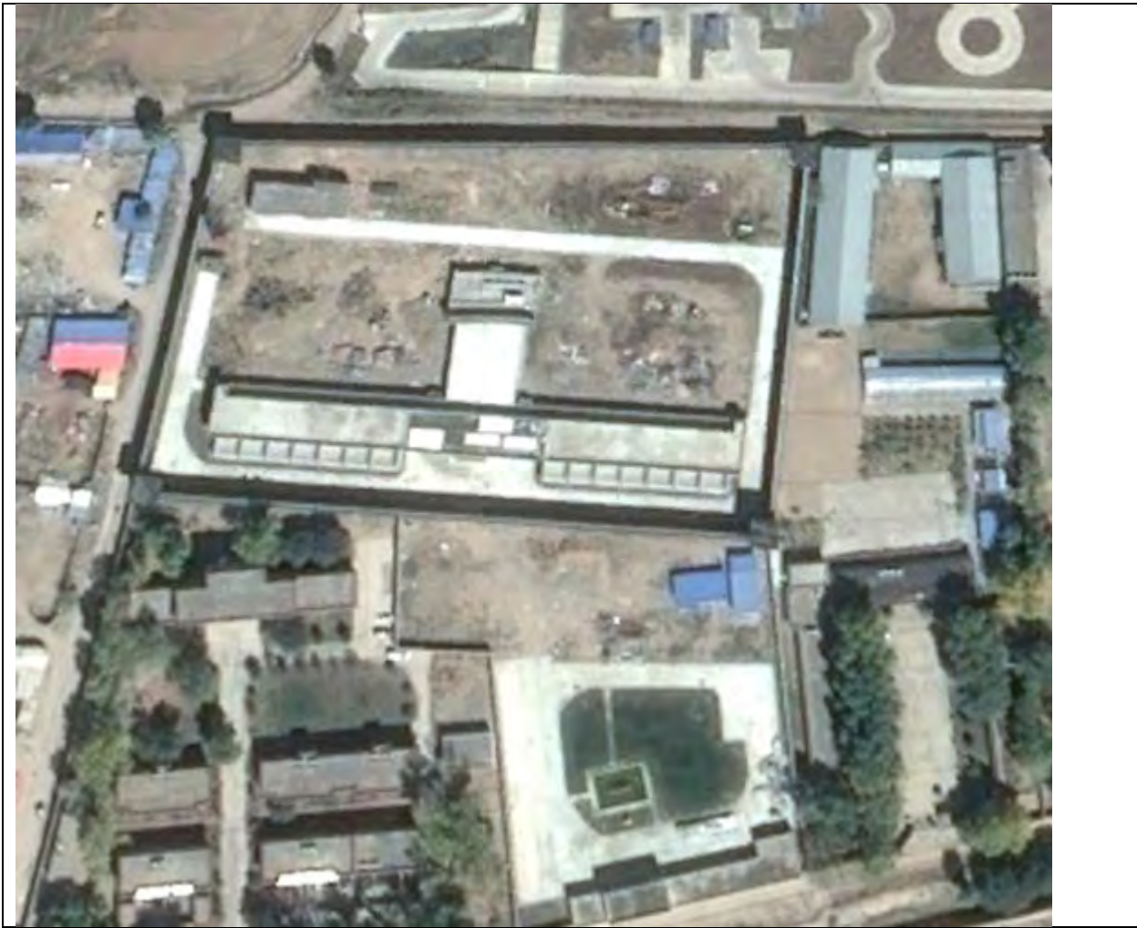
Image dated 2 nd October 2015 showing the facility complete or near completion.
