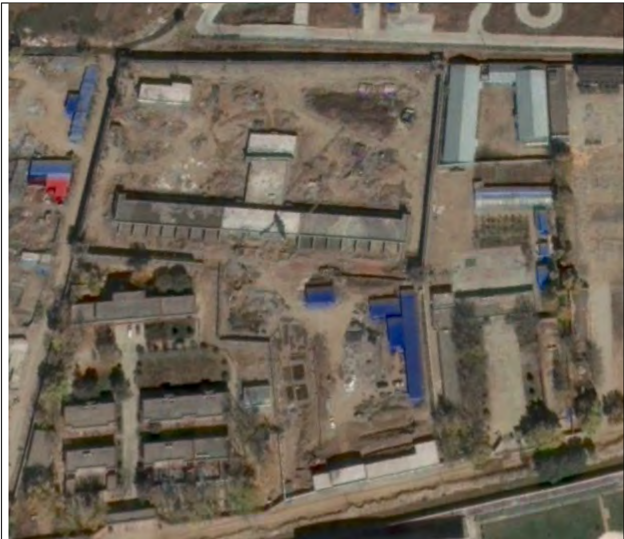
Image dated 20 th October 2014 showing the new facility being constructed.
