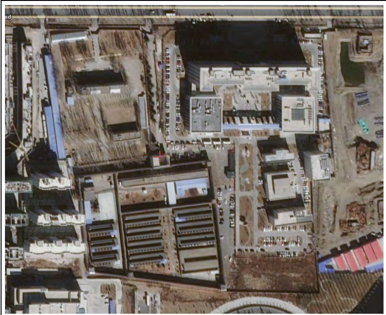
Figure 46 – Gutsa Detention Centre
