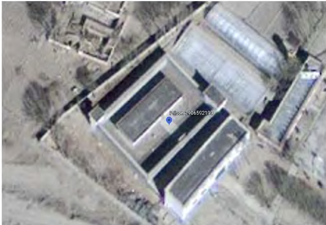
Figure 135 - Langkazi County Detention Center 2906592199
